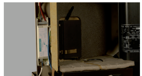
9 Position sensor in supply air stream (example)
